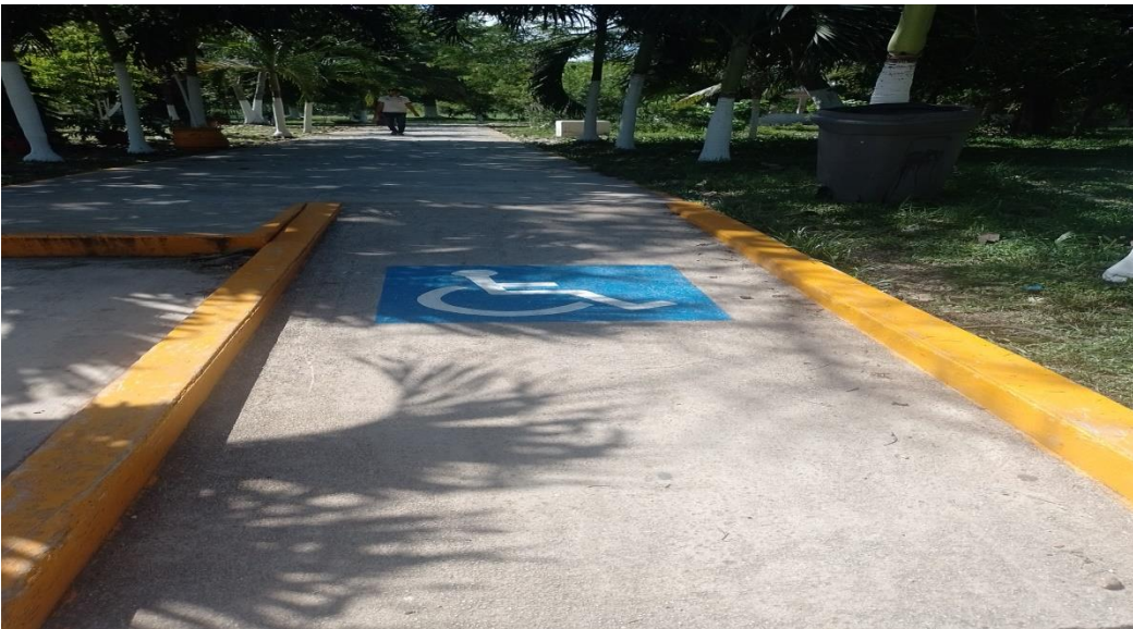
6. RAMPA RUMBO A CAFETERIA
